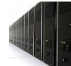
Data Center Services
